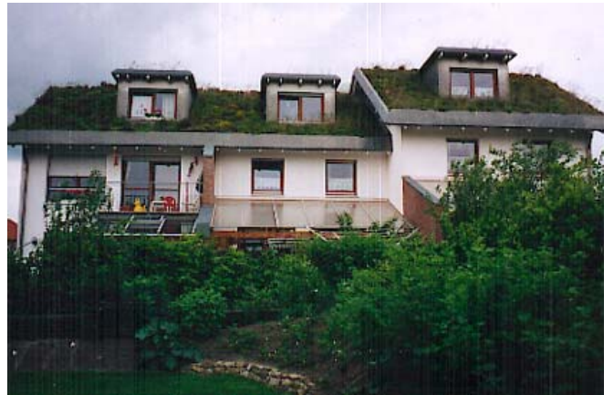
Vegetated Roof in Practice
