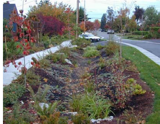
Example of a roadway bioswale in urban area
