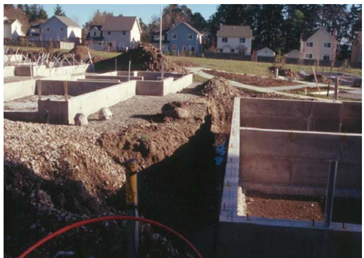
Low Impact Foundations Reduce Site Disturbance
