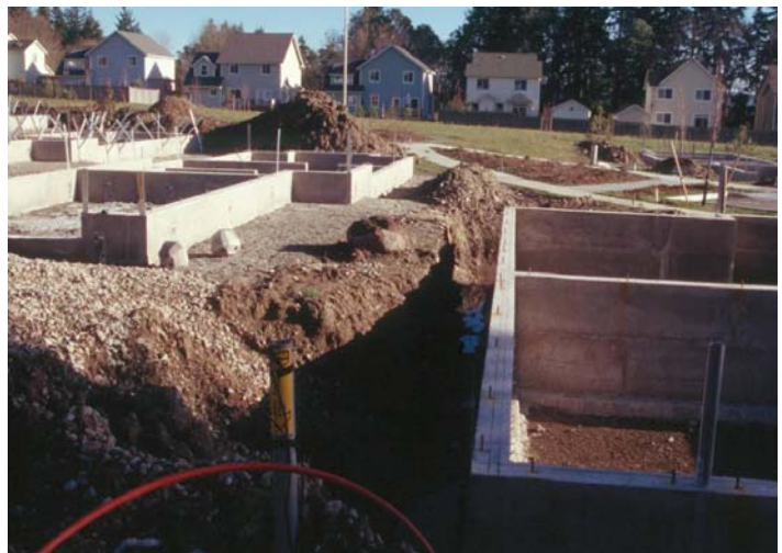
Low Impact Foundations Reduce Site Disturbance
