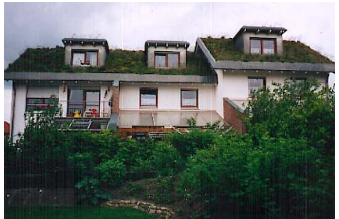
Vegetated Roof in Practice
